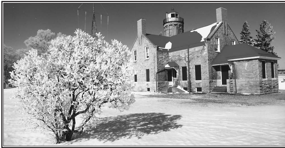
Old Mackinaw Point Lighthouse
